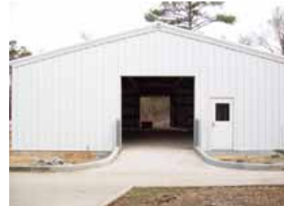
Irix Pharmaceutical Warehouse Florence, SC
